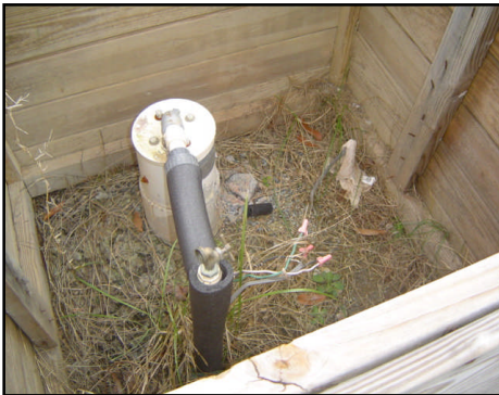
New Well Pump
